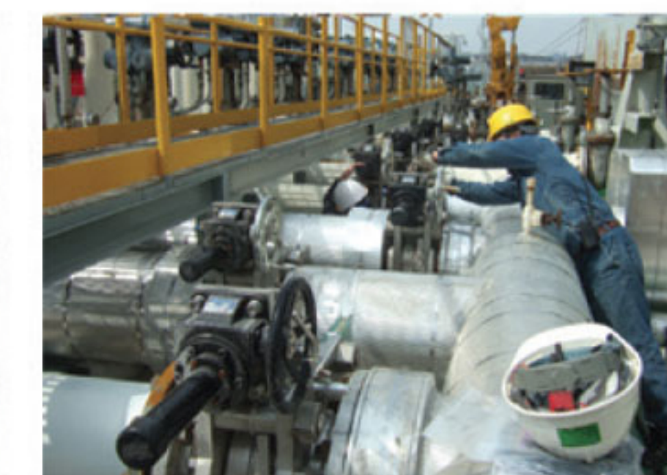
Loading Arm Construction
